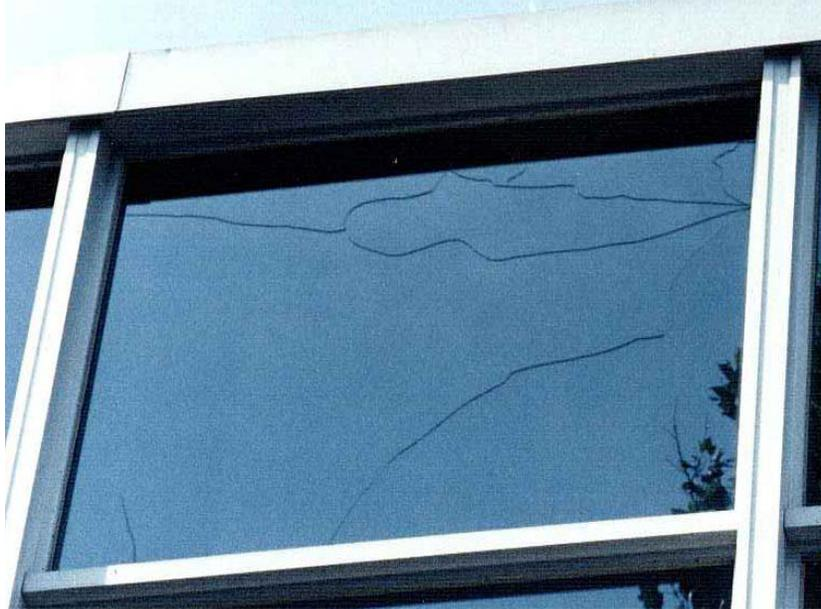
Typical, high stress fracture, originating at the right hand side. In this case insulation behind an annealed, heat absorbing glass and the shadow from an overhang caused excessive stress on a clean cut edge.
