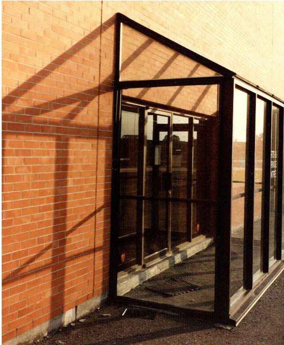
3. Inside corner reflections (where two curtain wall sections meet at a 90 deg angle, measured on the exterior, in plan view) cause increased temperature differences in glass when the heat from the grazing solar reflection of an adjacent glazing is added to the direct solar radiation.
